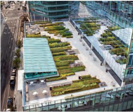
textured Tudor® finish provides slip resistant properties. Safer than gravel ballast, Hanover® pavers make roofs and plazas safe for pedestrians and simplify repairs.
