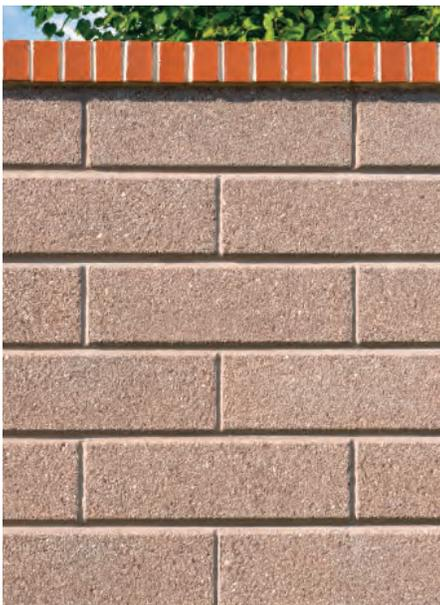
or lightweight product. Hanover's test results show high compressive strength, density and low water absorption qualities. Using cement as a binder, each product truly becomes Reconstructed Stone™.
