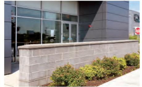
cleaned as necessary with masonry acidic cleaners and can be installed above or below grade. Reconstructed Stone™ Masonry units are made 3 5/8" thick and are available in five sizes.
