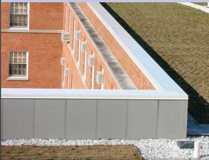
WallGUARD® panels are installed using specially designed galvanized steel mounting clips, which are included with each pallet of product. They can be installed in any weather, without the need for highly skilled labor. Due to the nature of their installation, WallGUARD® panels can be removed and reused when applicable.
