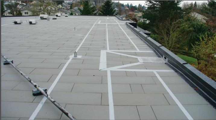
By simply reversing conventional design and placing the insulation above the membrane rather than below, the cause of many life shortening roofing problems can be eliminated. This unconventional arrangement of roofing material—roof deck, roof membrane, LightGUARD® or HeavyGUARD® ballasted roof insulation panels—is commonly referred to as the upside-down system, or Protected Membrane Roofing (PMR) system.
