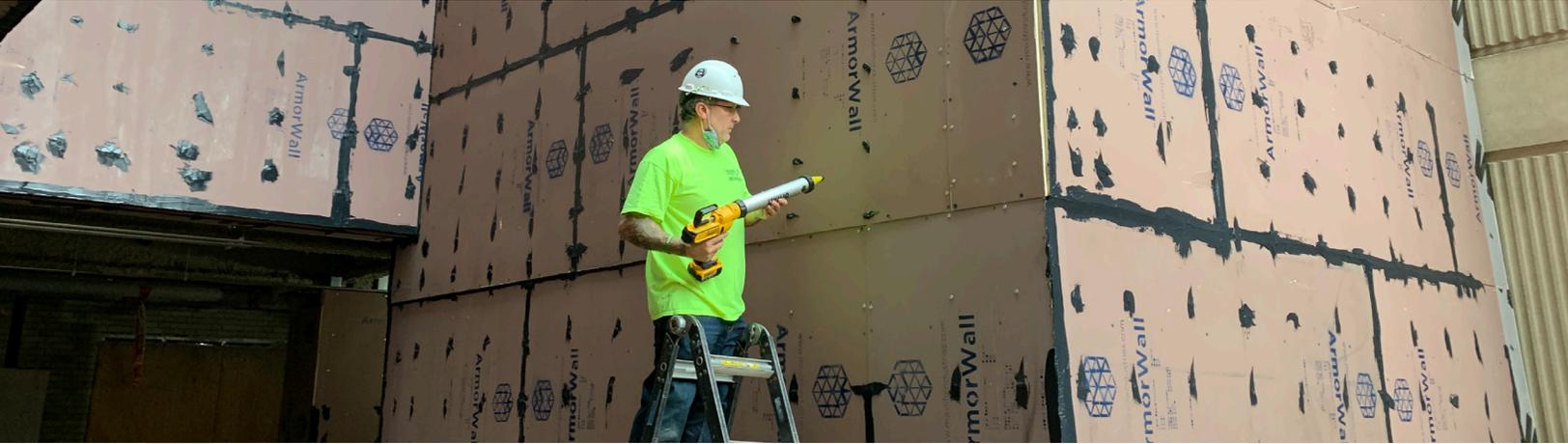
Due to the unique properties of the ArmorWall system and its components, it can be installed within various assemblies on many substrates, and at many locations that other systems cannot. Such diversity oftentimes can become confusing, so we at MaxLife have developed this Fastener Guide to aid the installer and designer in understanding the correct screw for each application.
