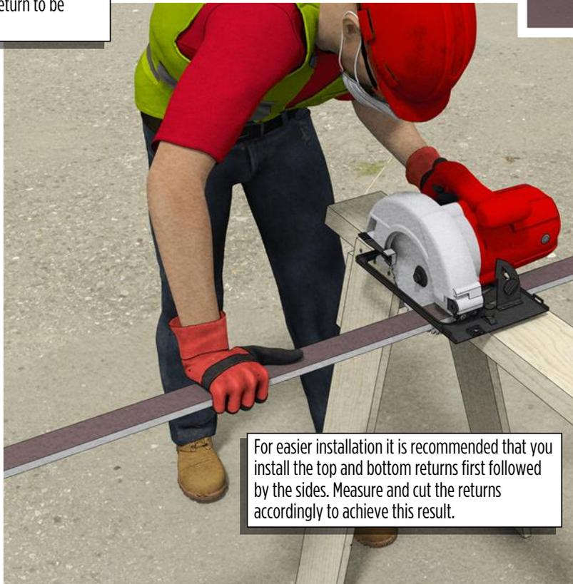
For easier installation it is recommended that you install the top and bottom returns first followed by the sides. Measure and cut the returns accordingly to achieve this result.
