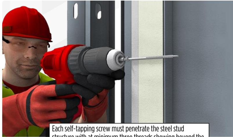
Each self-tapping screw must penetrate the steel stud structure with at minimum three threads showing beyond the metal surface.
