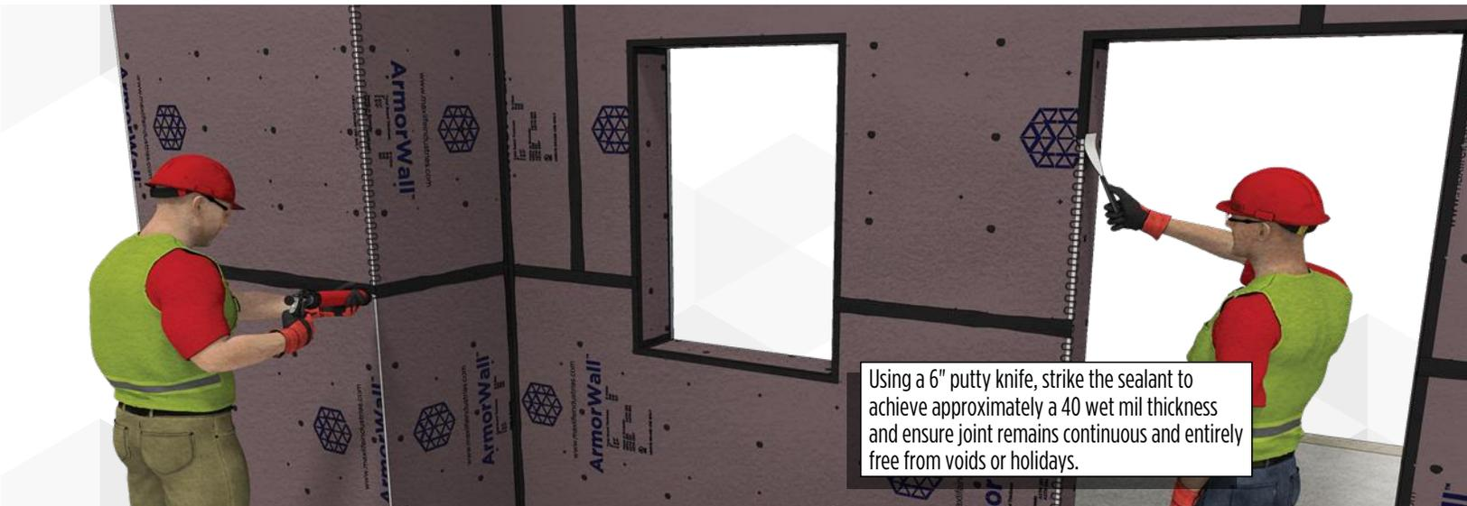
Using a 6" putty knife, strike the sealant to achieve approximately a 40 wet mil thickness and ensure joint remains continuous and entirely free from voids or holidays.
