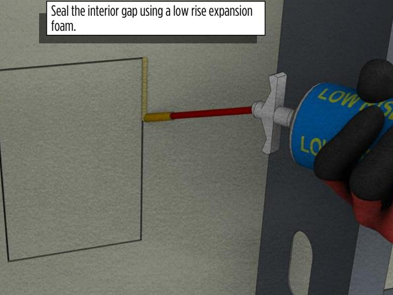
Seal the interior gap using a low rise expansion foam.
