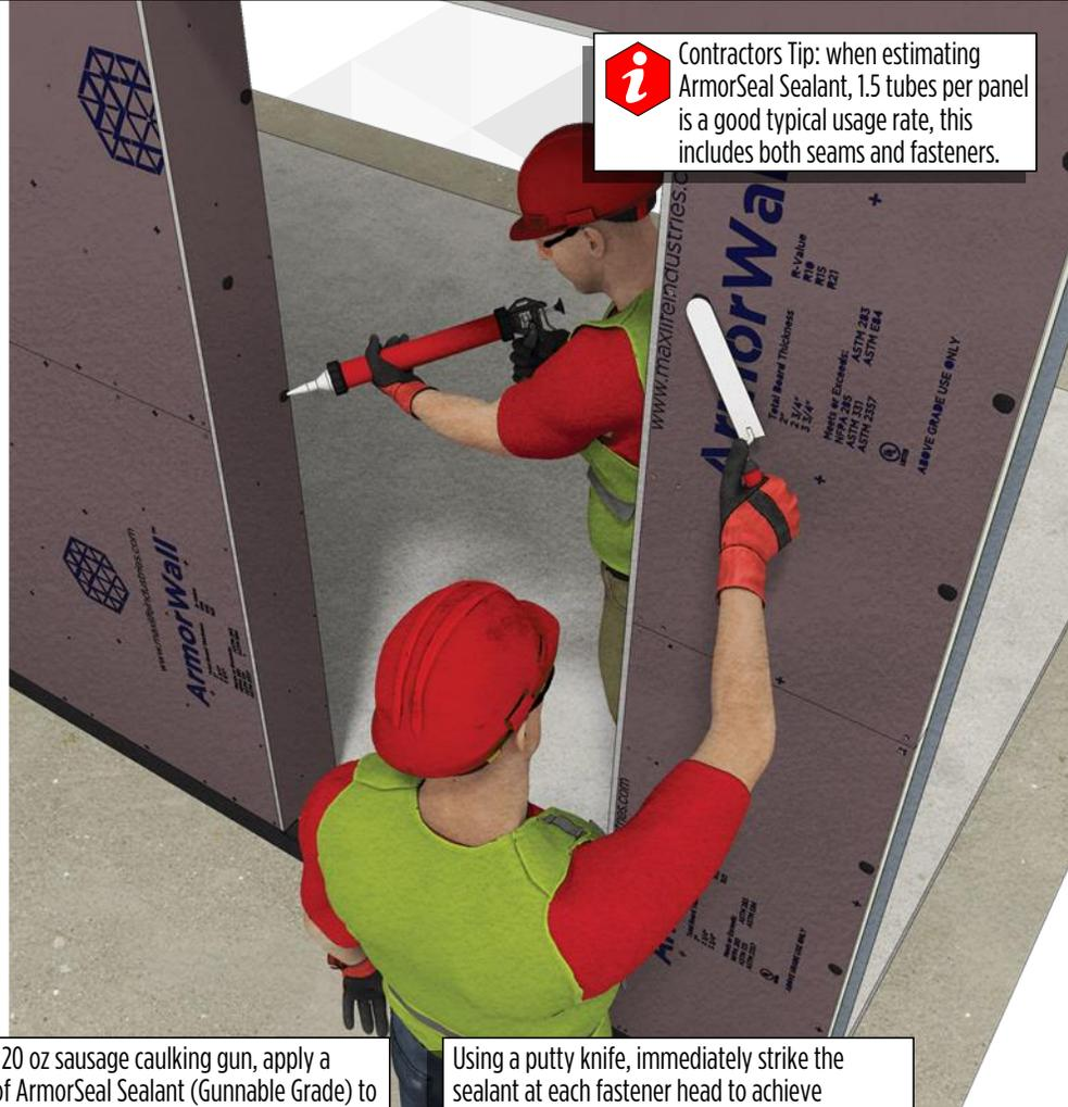
Using a 20 oz sausage caulkungun, apply a dollop of ArmorSeal Sealant (Gunnable Grade) to all exposed fastener heads with a sufficient amount to fully be sealed. Sealant should extend at least 1" around each fastener head.
