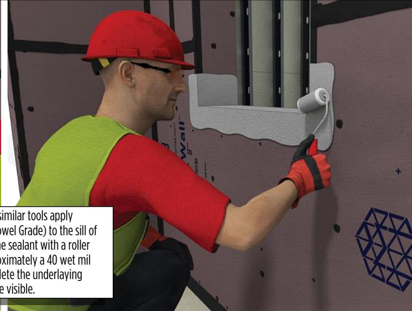
Using a putty knife or similar tools apply ArmorSeal Sealant (Trowel Grade) to the sill of the opening. Spread the sealant with a roller brush to achieve approximately a 40 wet mil thickness. When complete the underlying substrate should not be visible.
