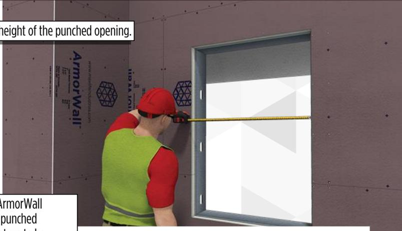
Panel depth returns require the ArmorWall panels to be cut 1/2" short of the punched opening allowing the 1/2" thick return to be installed flush to the opening.
