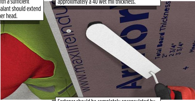
Fastener should be completely encapsulated by ArmorSeal Sealant forming an airtight seal.
