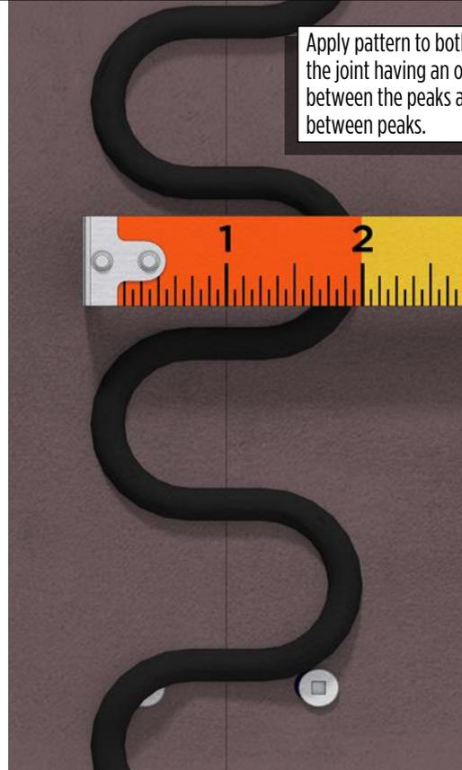
Apply pattern to both surfaces which comprise the joint having an overall distance of 2" between the peaks and valleys and 2 1/2" between peaks.
