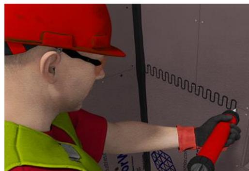
Using a 20 oz sausage caulkung gun, apply ArmorSeal Sealant (Gunnable Grade) in zig zag pattern across entire horizontal and vertical joint lines. Field seams receive 1" of continuous bead on each panel surface face to create a minimum 2" wide seam joint. Strike as before.
