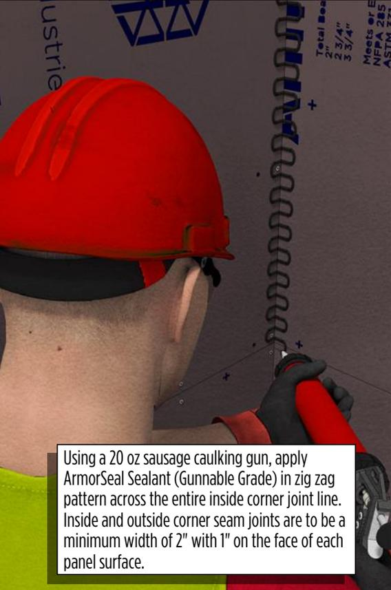
Using a 20 oz sausage caulkung gun, apply ArmorSeal Sealant (Gunnable Grade) in zig zag pattern across the entire inside corner joint line. Inside and outside corner seam joints are to be a minimum width of 2" with 1" on the face of each panel surface.
