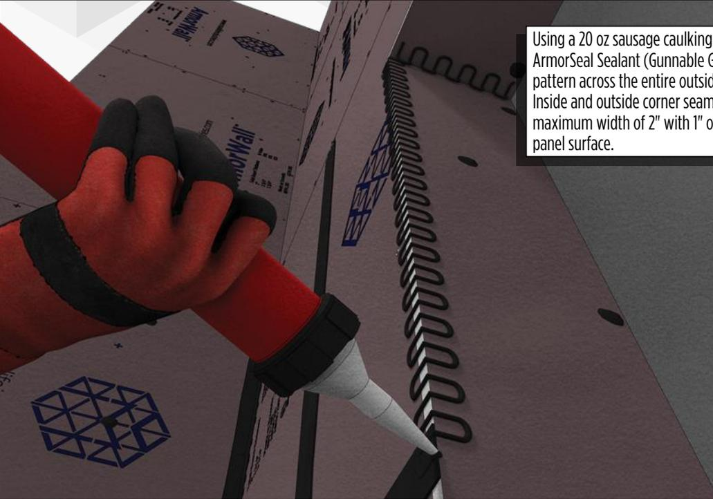
Using a 20 oz sausage caulking gun, apply ArmorSeal Sealant (Gunnable Grade) in zig zag pattern across the entire outside corner joint line. Inside and outside corner seam joints are to be a maximum width of 2" with 1" on the face of each panel surface.
