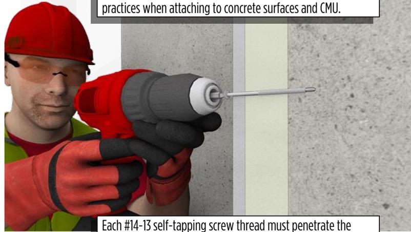
Each #14-13 self-tapping screw thread must penetrate the concrete structure a minimum of 1".
