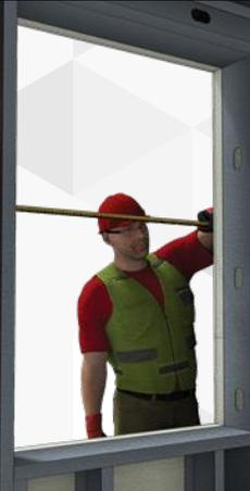
For easier installation it is recommended that you install the top and bottom returns first followed by the sides. Measure and cut the returns accordingly to achieve this result.
