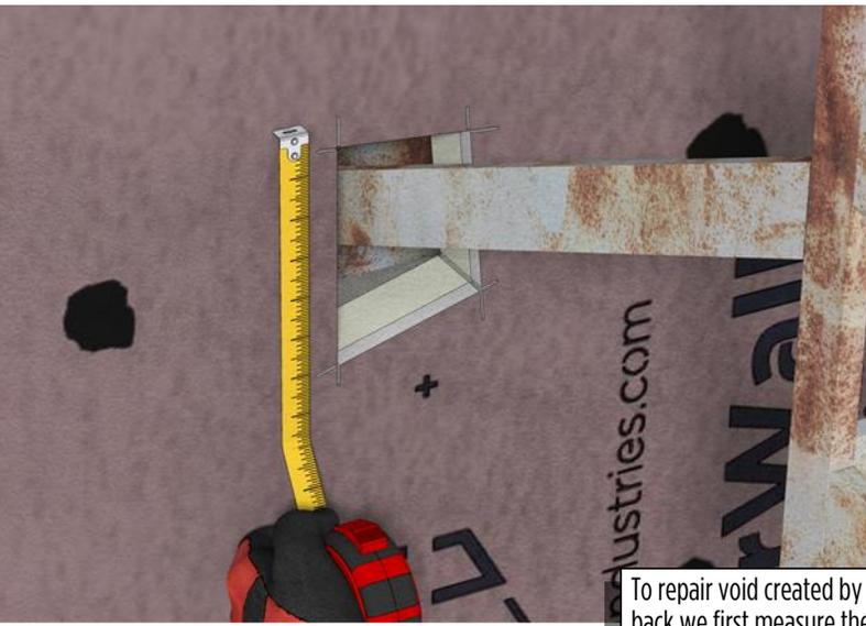
To repair void created by the penetrating tie-back we first measure the overall dimensions vertically and horizontally. Measure off and cut any available, undamaged, and clean ArmorWall material and cut it to size.
