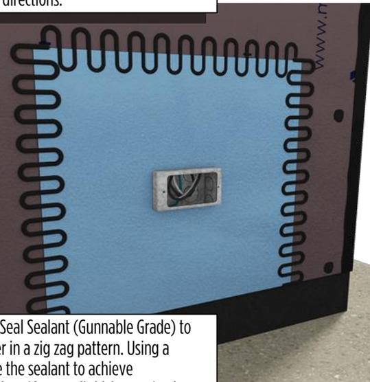
Allow full cure duration of the ArmorSeal target patch and apply ArmorSeal Sealant (Gunnable Grade) to the perimeter in a zig zag pattern. Using a trowel, strike the sealant to achieve approximately a 40 wet mil thickness.
