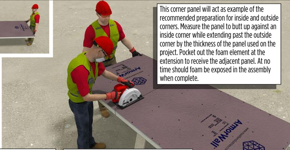
This corner panel will act as example of the recommended preparation for inside and outside corners. Measure the panel to butt up against an inside corner while extending past the outside corner by the thickness of the panel used on the project. Pocket out the foam element at the extension to receive the adjacent panel. At no time should foam be exposed in the assembly when complete.
