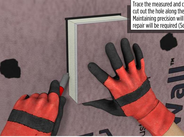
Trace the measured and cut panel and carefully cut out the hole along the traced marking. Maintaining precision will determine which gap repair will be required (See pages 35 and 36).
