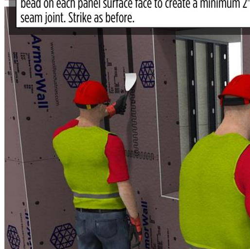
**i** Contractors Tip: when estimating ArmorSeal Sealant, 1.5 tubes per panel is a good typical usage rate, this includes both seams and fasteners.
