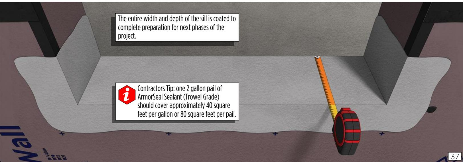
The entire width and depth of the sill is coated to complete preparation for next phases of the project.
