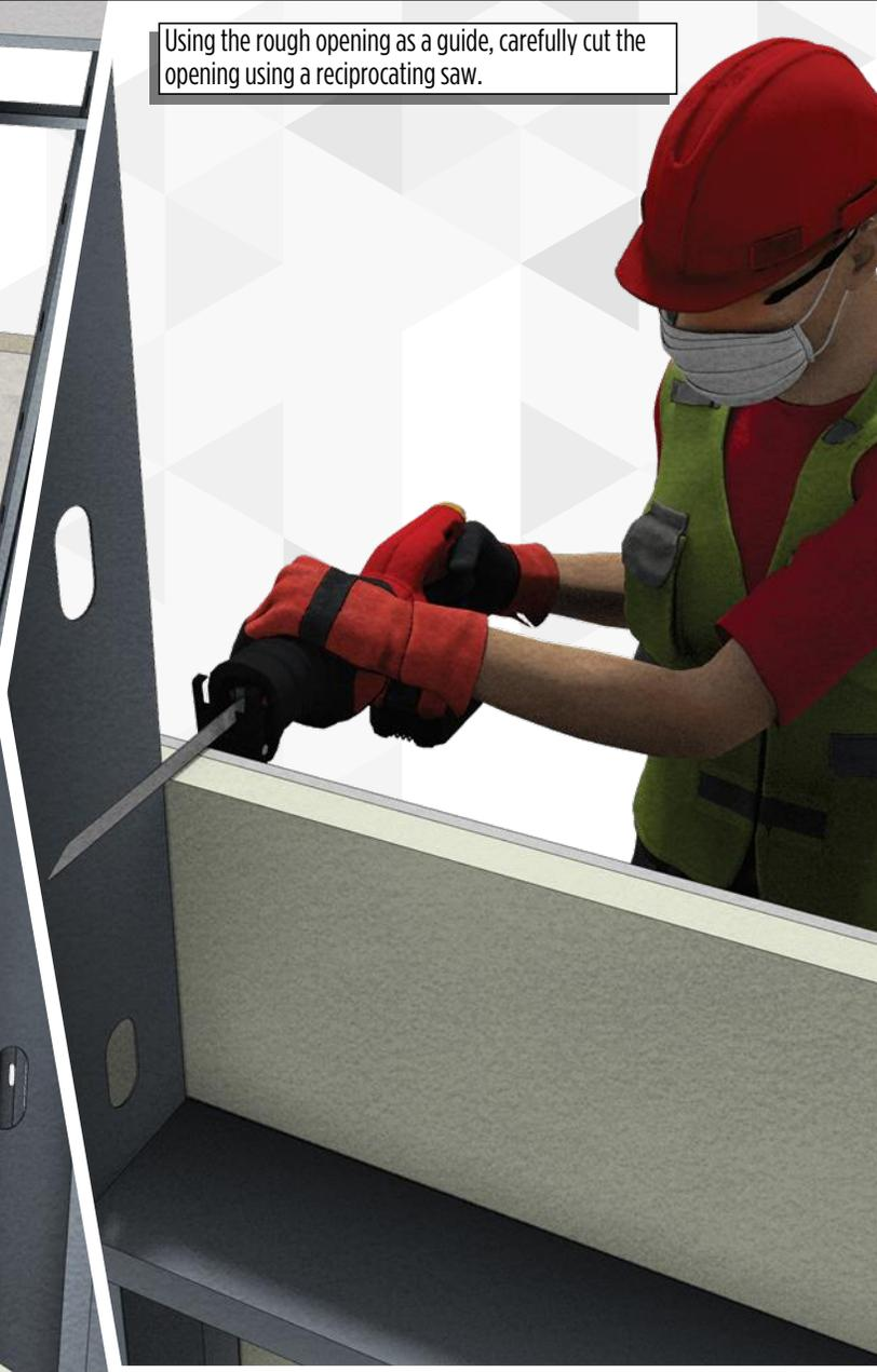
Cut away the extra panel at the door punched opening, again using the opening as the guide.
