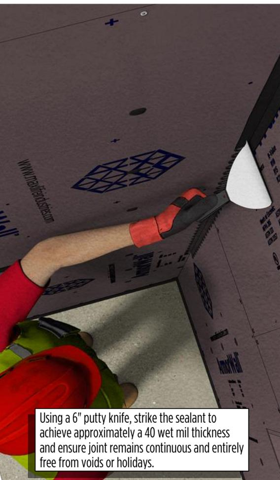
Using a 6" putty knife, strike the sealant to achieve approximately a 40 wet mil thickness and ensure joint remains continuous and entirely free from voids or holidays.
