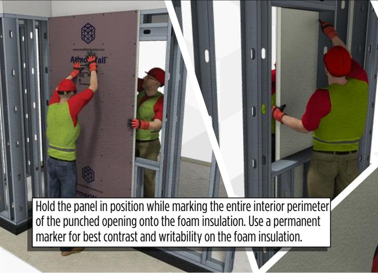
Hold the panel in position while marking the entire interior perimeter of the punched opening onto the foam insulation. Use a permanent marker for best contrast and writability on the foam insulation.
