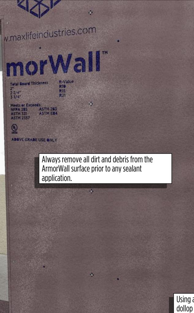
Always remove all dirt and debris from the ArmorWall surface prior to any sealant application.
