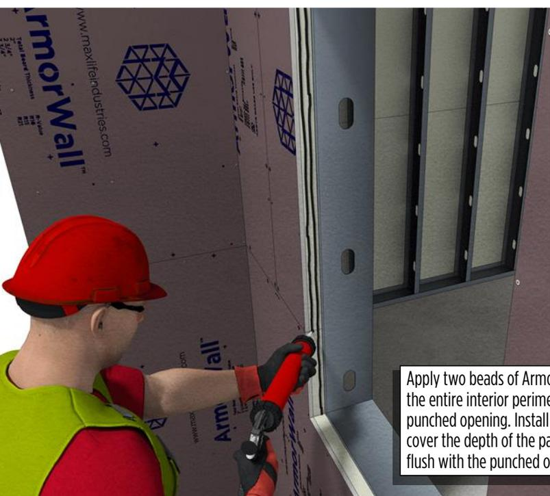
Apply two beads of ArmorSeal Sealant around the entire interior perimeter panel surface at the punched opening. Install the pre-cut returns to cover the depth of the panel and ensure each sits flush with the punched opening.
