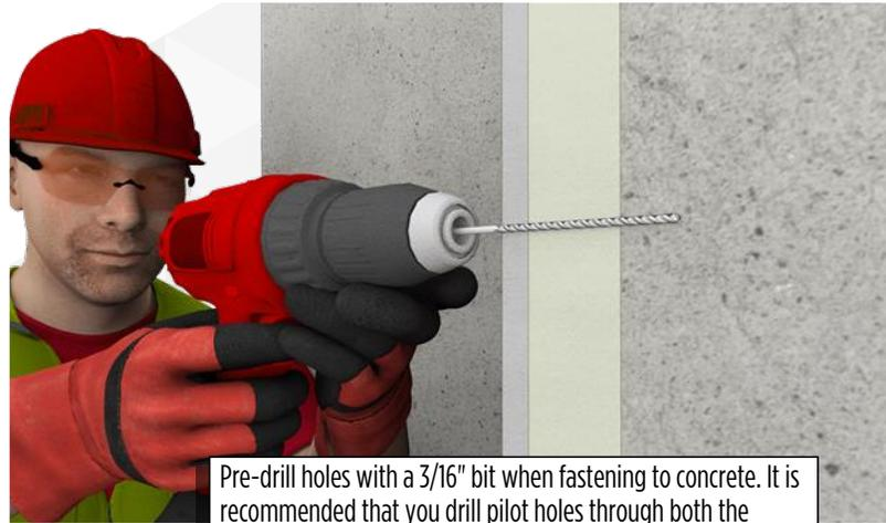
Pre-drill holes with a 3/16" bit when fastening to concrete. It is recommended that you drill pilot holes through both the panel and concrete. Follow standard fastener manufacturer practices when attaching to concrete surfaces and CMU.
