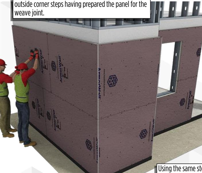
Using the same steps as the first row of panels continue to install ArmorWall up the structure.
