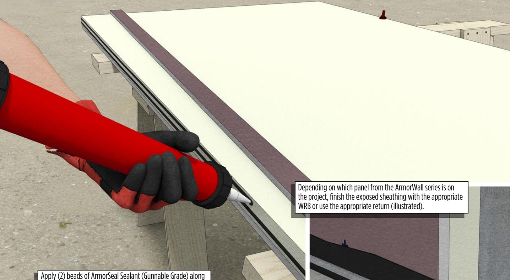
Apply (2) beads of ArmorSeal Sealant (Gunnable Grade) along the edge of the panel and adhere the ArmorBoard Plus Return.
