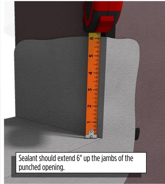
Sealant should extend 6" up the jambs of the punched opening.
