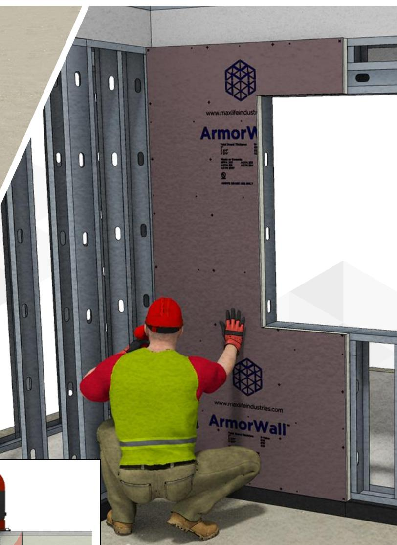
Install ArmorWall panels from the center working outwards to help alleviate any possible cupping that could have resulted from transport.
