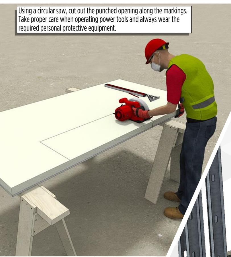
Using a circular saw, cut out the punched opening along the markings. Take proper care when operating power tools and always wear the required personal protective equipment.
